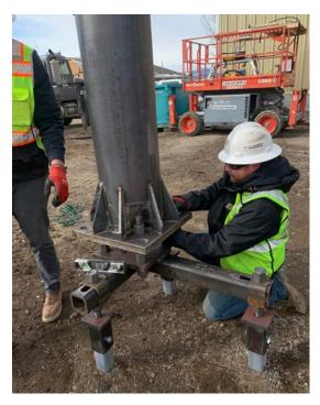
4. Structure attached to adapter component
