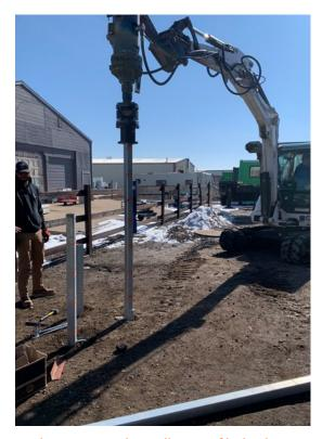
1. Alignment and installation of helical piers
