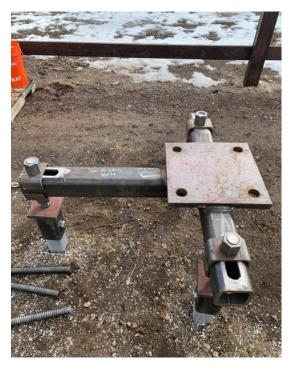
3. Adapter component connected to pier caps
